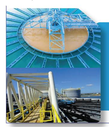
HRSCC systems rapidly mix and flocculate solids with chemical coagulants, producing clear effluent and dense sludge. Enhanced HRSCC systems offer improved performance and higher treatment capacities.
