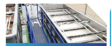
DAF systems remove oil, grease, and suspended solids from water by dissolving air in the water under pressure and then releasing it at atmospheric pressure, causing contaminants to float to the surface for removal.
